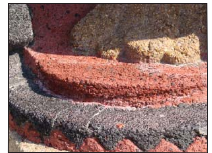
Detail of Minisa Bridge
