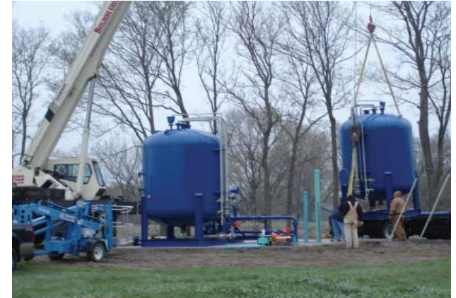
Installation of carbon units for treating contaminated groundwater.
