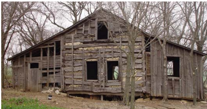
The original Heller Cabin before restoration
