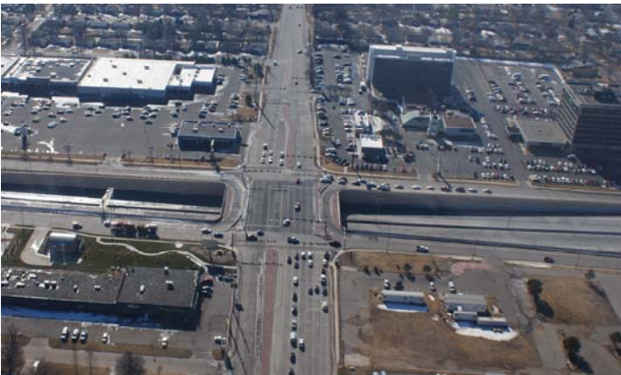
Kellogg/Rock interchange project
