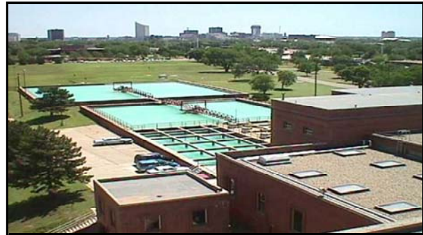
The water treatment plant at Sim Park.
